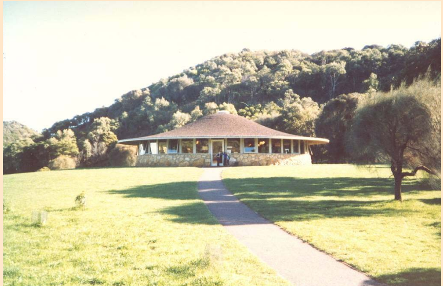
The Worn Gundidj Visitor Centre, designed by Robin Boyd in 1962.
